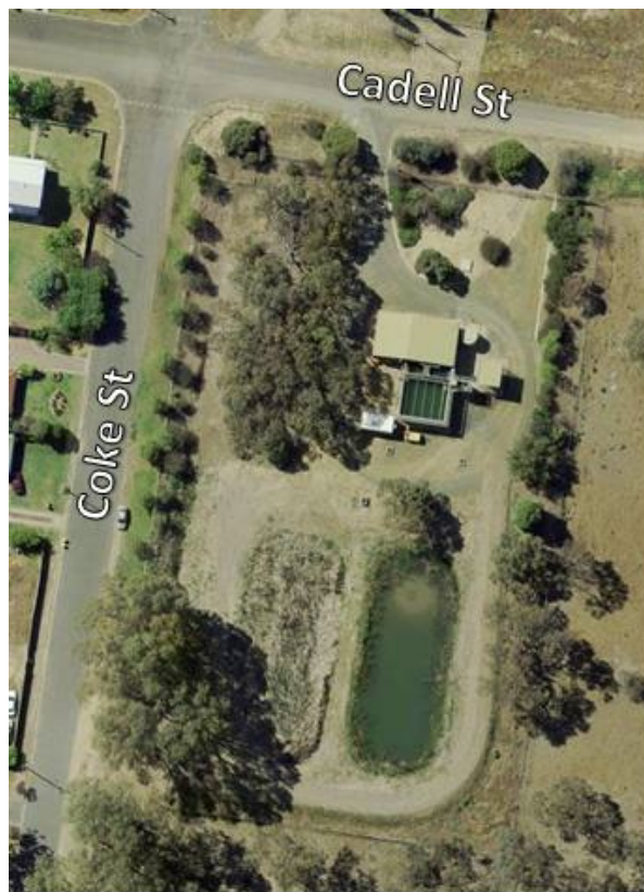
Figure.1.3 Hay Water Treatment Plant
